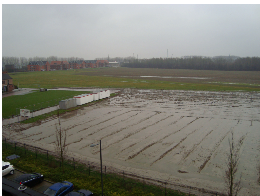
Brede School fase bouwput
